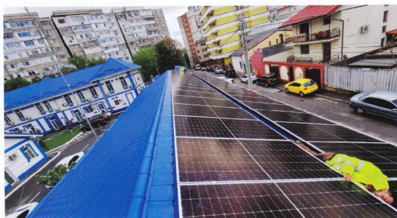
Fig. 26. Panouri fotovoltaice sediul APA CANAL S.A. Galați / Photovoltaic panels at APA CANAL S.A. Galati headquarters
